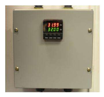
When properly connected, the Nitrox Controller will <u>only</u> open the oxygen control valve if the compressor is running.
