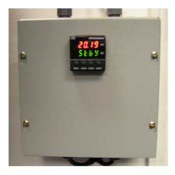
When the Nitrox Controller is the **Standby** mode, it will stop blending Nitrox, close the oxygen control valve, and silence any alarms.
