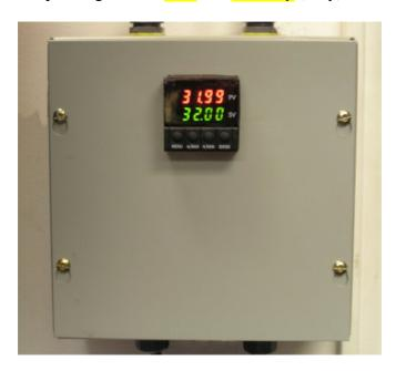
When the Nitrox Controller is in the **Standby** mode, to place it into the **Run** mode, press the **Enter** button once.
